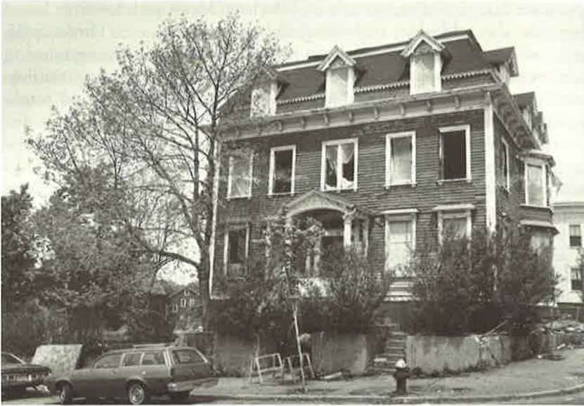
Figure 20. Villa Excelsior, 1208 Doyle Street, Providence, Rhode Island, May 1983, The Women's Development Corporation, architects and developers. One of the abandoned houses targeted for substantial rehabilitation for low-income single mothers by the Women's Development Corporation. Photograph courtesy The Women's Development Corporation.
